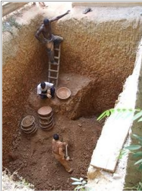
John, Francis and Lawrence digging the cess pit
